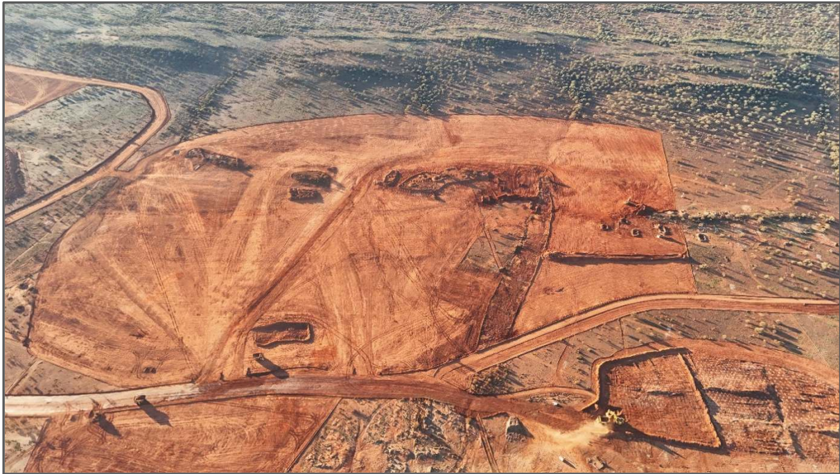
Figure 1: Cue open pit mining commencement
