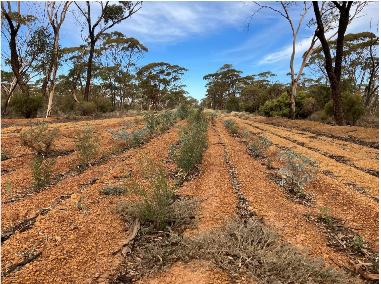
Figure 5: Photo of Warrachuppin road rehabilitation March 2024.
